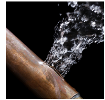
STOP PINHOLE LEAKS
