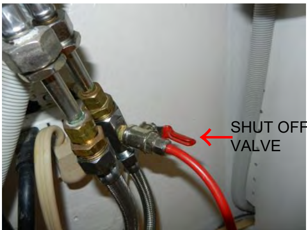
Filter red tube connection to separate valve.
